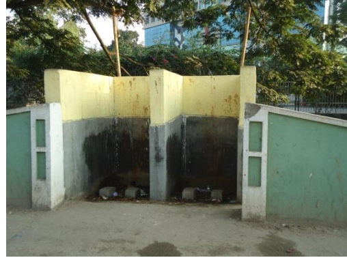
Newly constructed open
