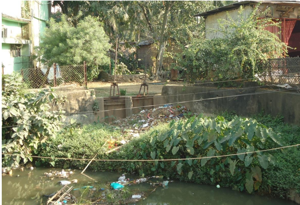
Figure 8-9 The closed sluice gate of Bahini at Nutan Bazaar
