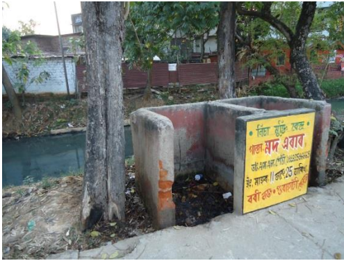
Open toilet block along Bahini River toilet block
